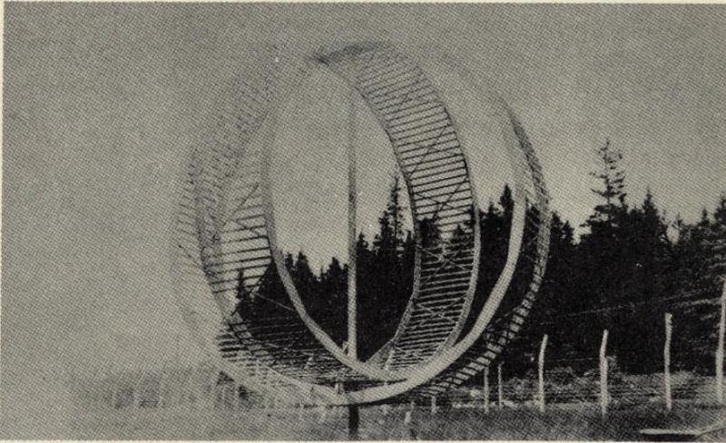
The Pickard directional loop receiving antenna, Otter Cliffs.
